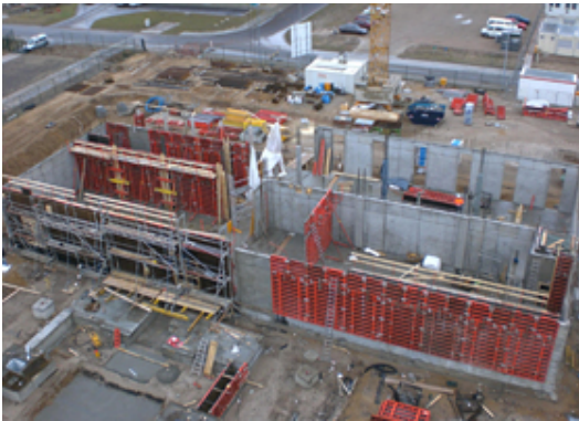
Construction of the Bitterfeld site
